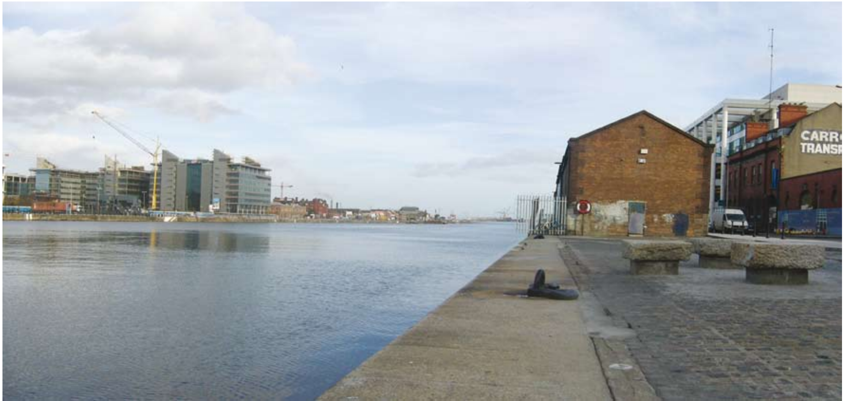
The BJ Marine warehouse on Sir John Rogerson's Quay - existing situation
